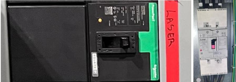
The MSC controller is supplied from a 200A circuit breaker with 3/0 CU conductors & are landed on a 150A breaker / disconnect inside the enclosure. This is compliant with NEC. The MSC controller then feeds (3) sub-panels. All feeds have appropriate over current protection
